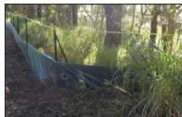
TREE PROTECTION & EROSION FENCE
