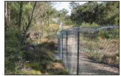
FAUNA EXCLUSION FENCING
