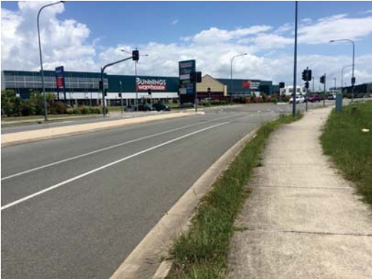
4 Approx. 1.8m wide concrete path and 500mm wide grass area between the kerb and the path
