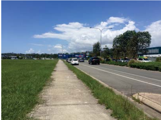
3 Approx. 2.5m wide concrete path and 900mm wide grass area between the kerb and the path
