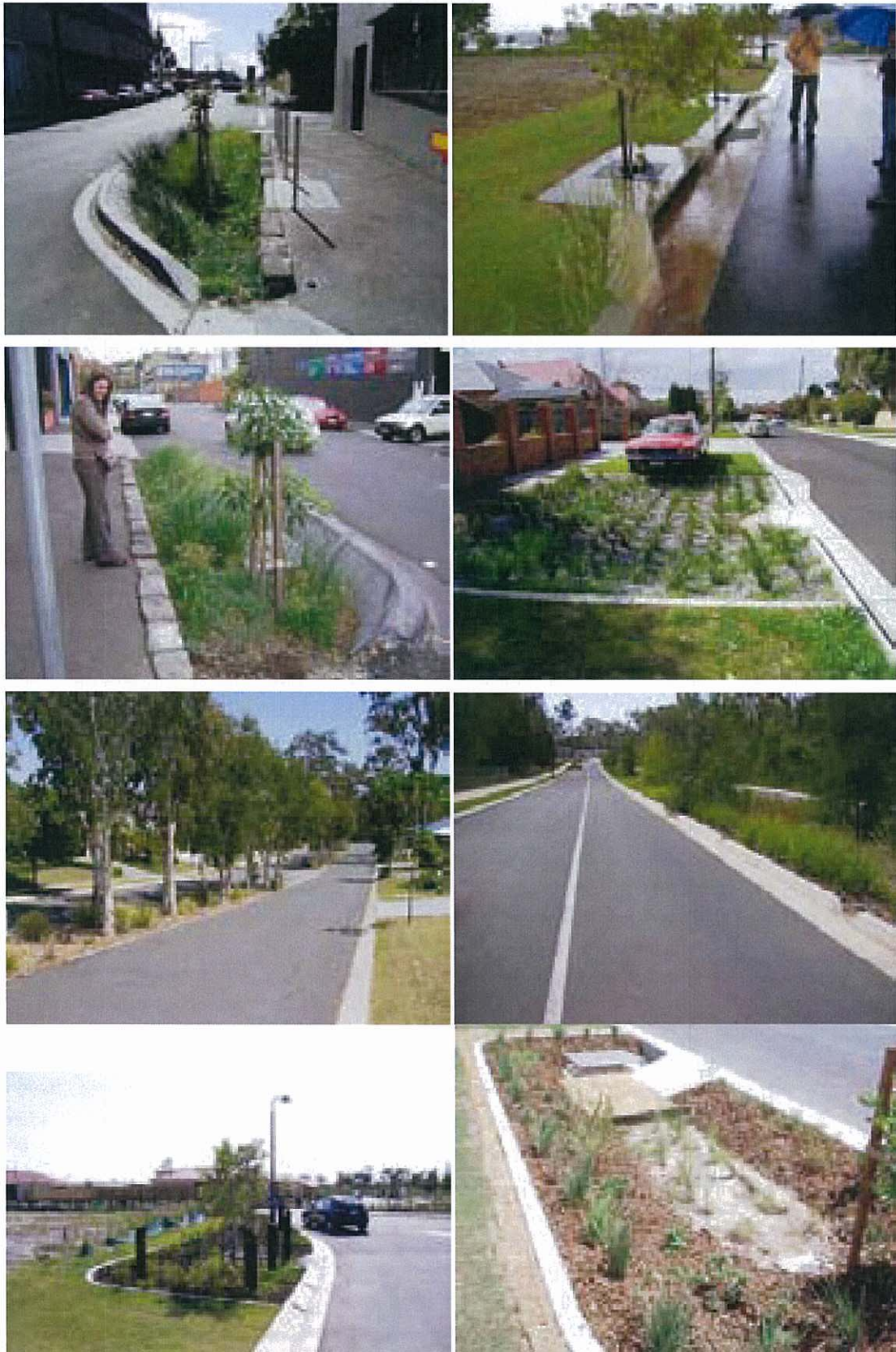
Figure 3-8 Examples of Streetscape Bioretention
