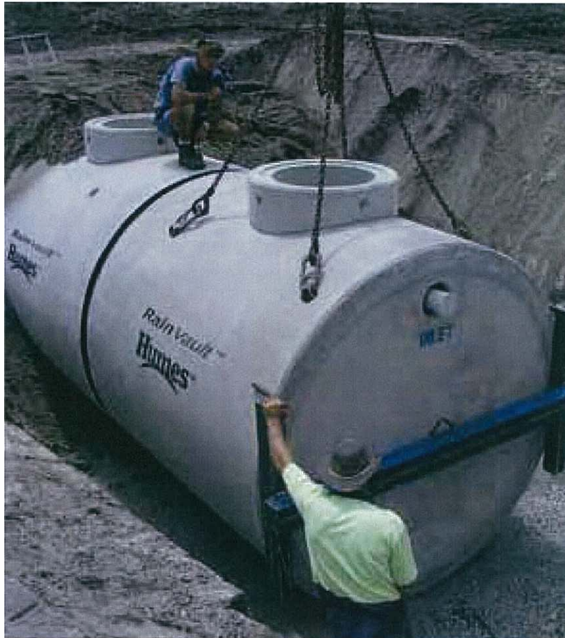
Figure 3-10 Installation of an Underground Stormwater Harvesting Tank
