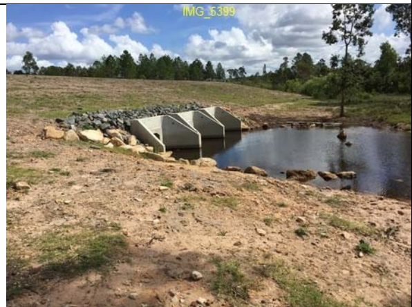
CH600 Interim flood bund 16-INT (downstream side). Post-civil works so minimal established vegetation evident.
