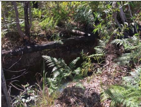
CH900-1000 narrow incised low flow channel (1m wide to 0.75m deep) alternating with grassed broad sheet flow area, small pockets of scour pool, generally goof vegetation cover outside low flow channel.
