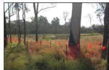
SIGNIFICANT TREE PROTECTION FENCING
