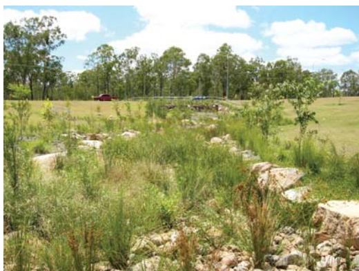
Plate 6.2 – Typical Bio-Retention System
