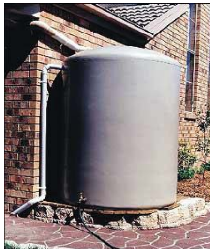
Plate 6.1 – Typical Rainwater Tank
