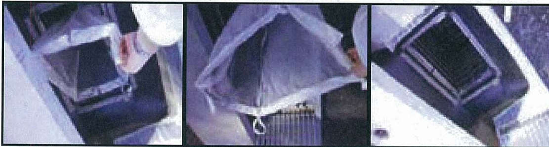
Figure 3-7 Pictures of Gully Baskets and Filter Mesh Installation
