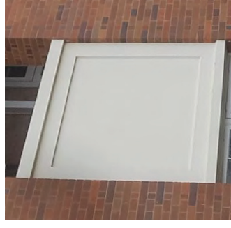
PT 4 PAINT TO LEVEL 1 UPSTANDS - TOWERS NEW PAINT TO MATCH EXISTING
