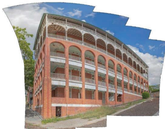
Figure 15 – Example of Façade Elevation Composite Panorama Photograph
