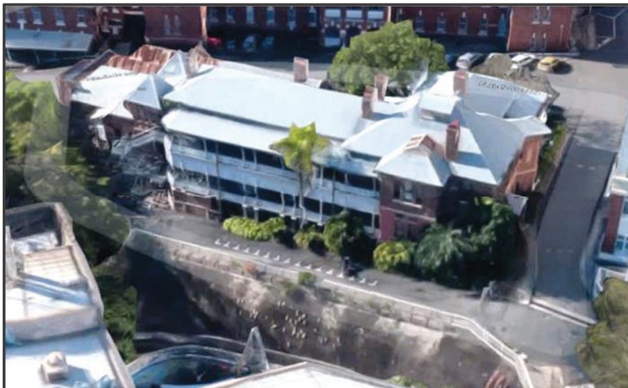
Figure 11 – Lady Norman Building
