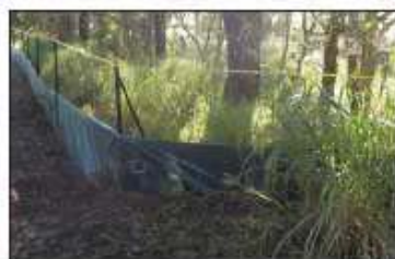
TREE PROTECTION & EROSION FENCE
