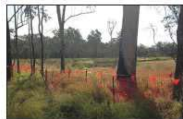
SIGNIFICANT TREE PROTECTION FENCING
