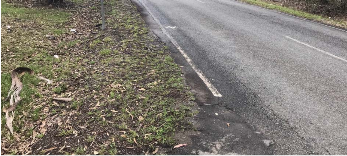
Figure 2-9 Faded linemarking and missing signage at intersections
