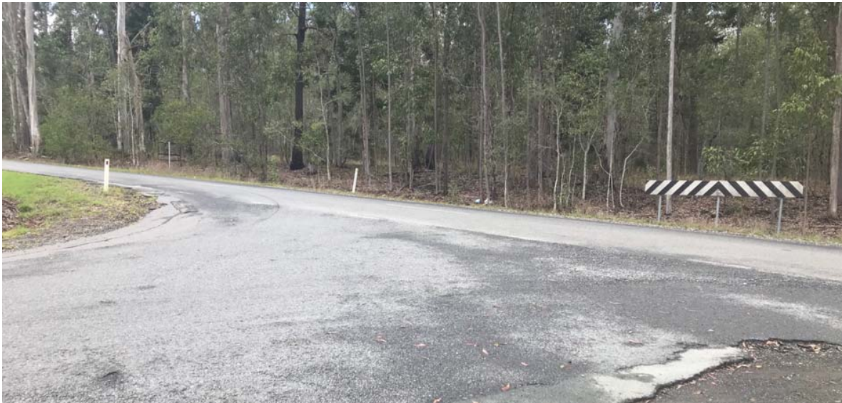
Figure 2-9 Faded linemarking and missing signage at intersections
