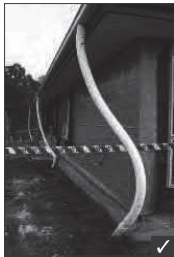
Temporary roof water connection
