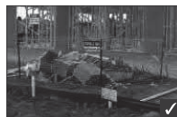
One way to properly store building waste
