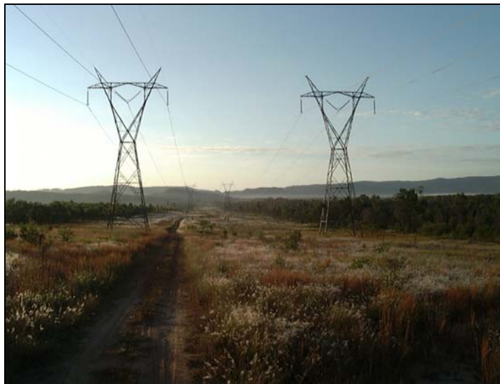
PLATE 1: GENERAL VIEW OF THE SITE LOOKING SOUTHEAST FROM NEAR THE INTERSECTION OF THE POWER LINES AND WATERFORD TAMBORINE ROAD.
