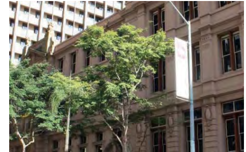
The Printery Building and existing streetscape
