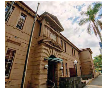
Former DPI Building entrance
