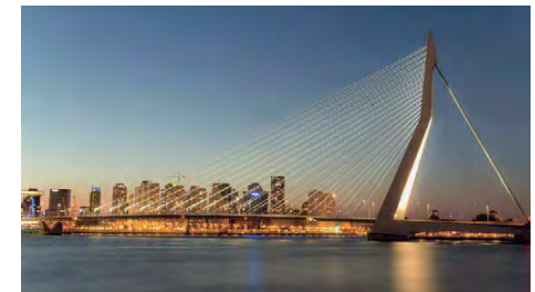
Bridge elements can be important points of visual reference and wayfinding
