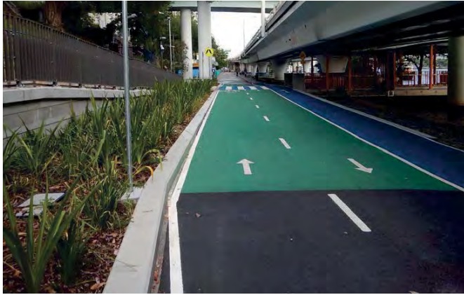
Figure 5.37: North Quay Existing Bikeway Conditions
