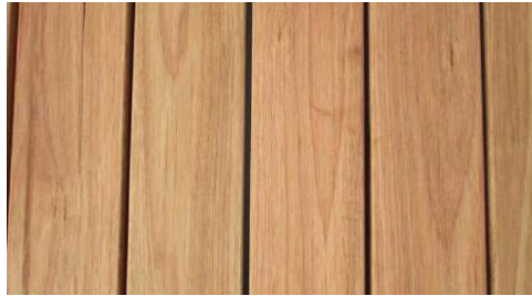
TM01 | TIMBER CLADDING
