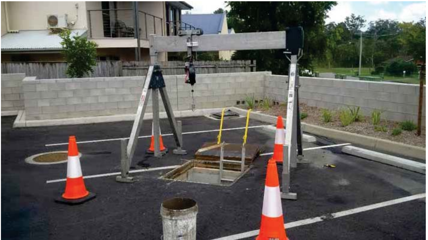
Figure 4. SPEL Filter install set-up
