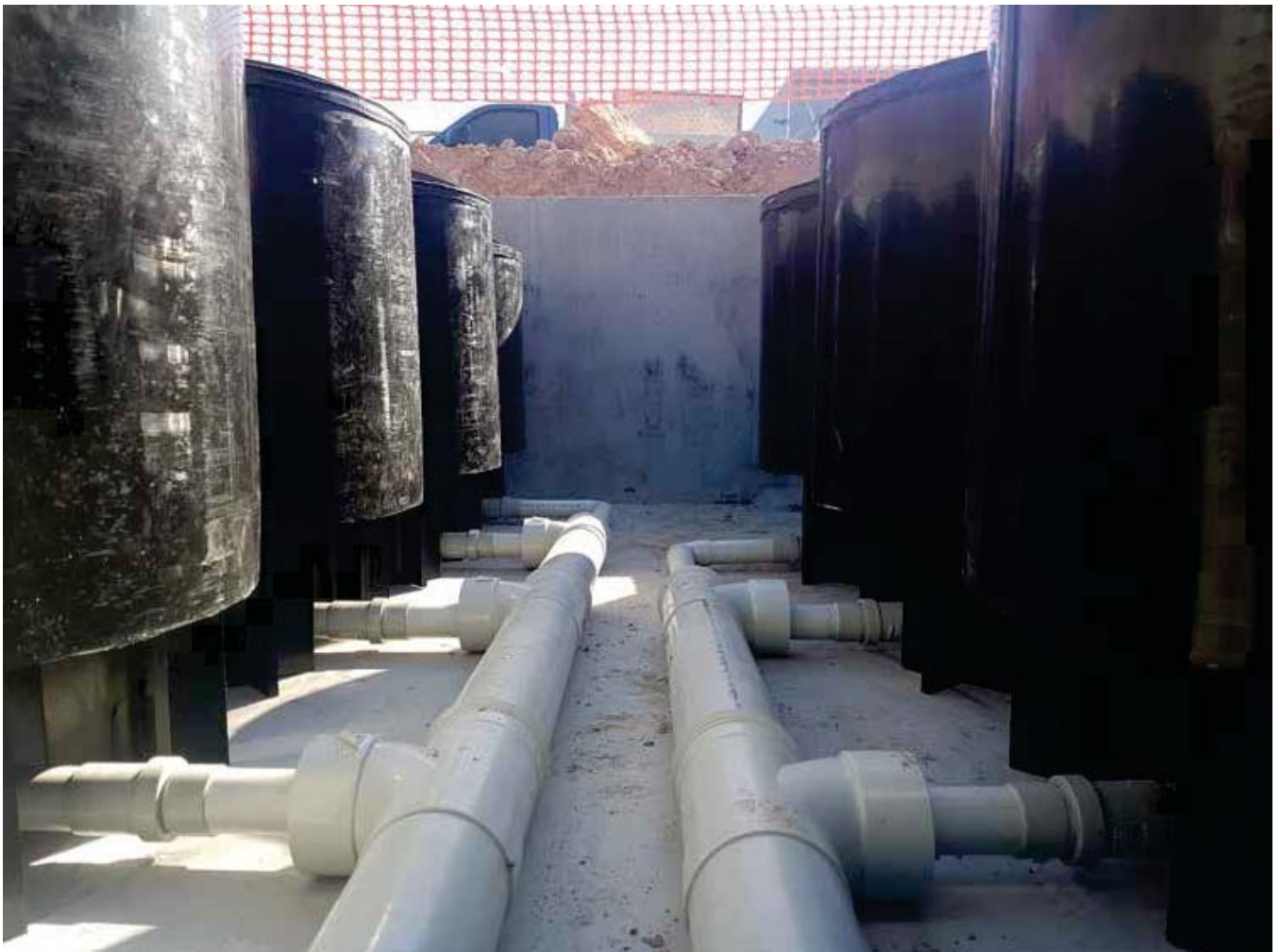
Figure 2. SPEL Filter install
