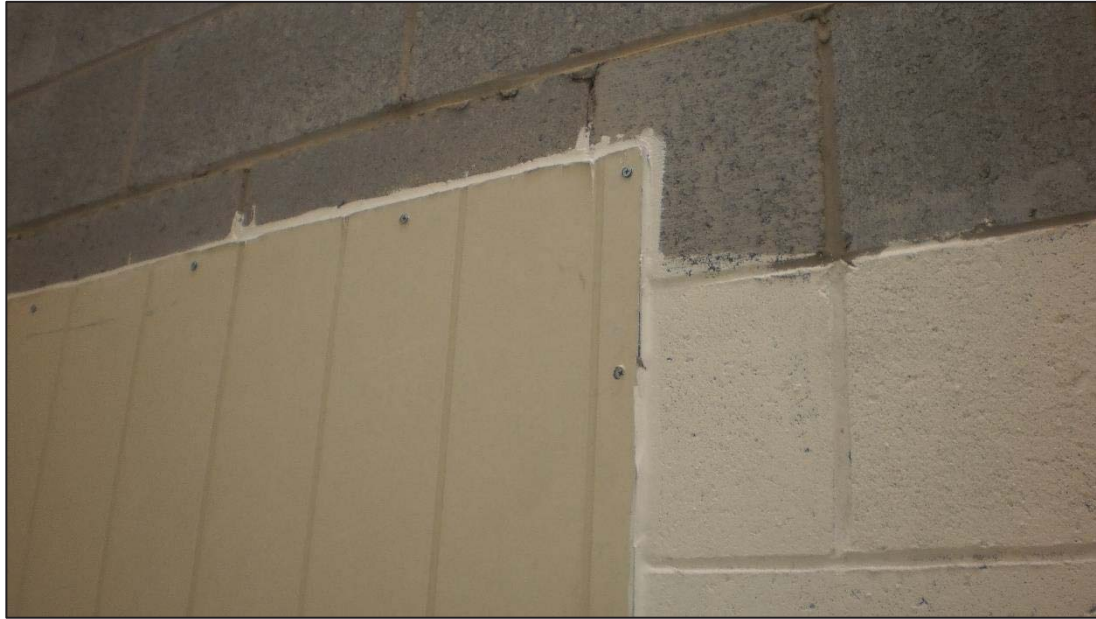
Photo 4: Showing the acoustic treatment applied to seal off the existing louvres
