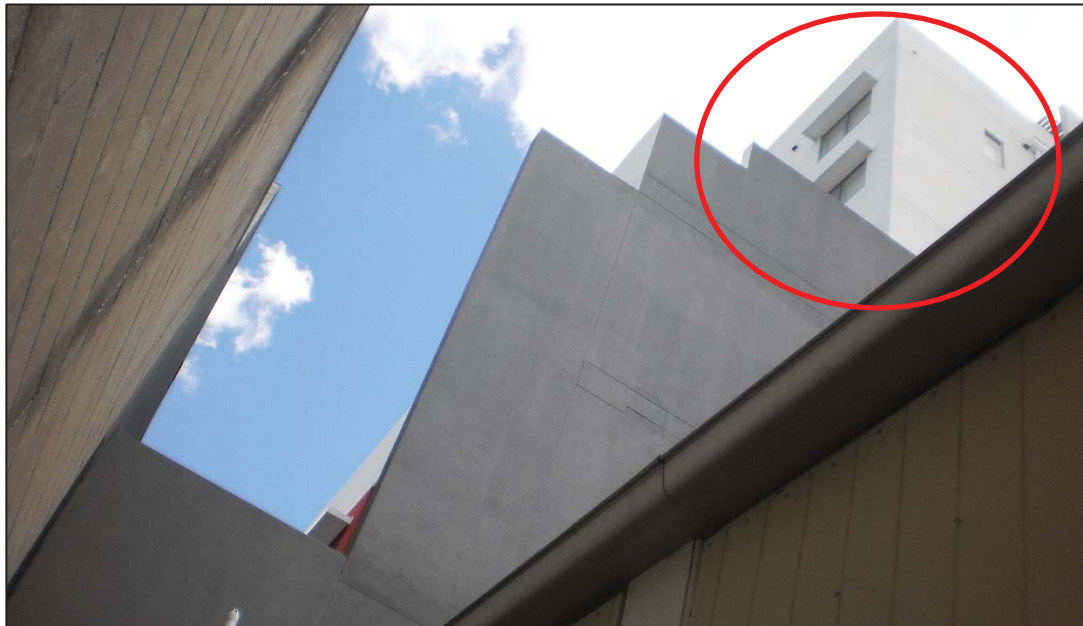
Photo 5: Showing the residential facades most exposed to potential noise breakout
