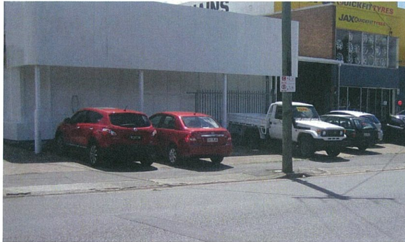
Figure 3.3b: Existing access arrangement (62-66 Abbotsford Road)
