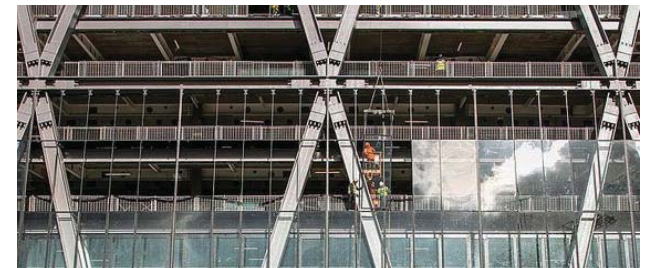
CONSTRUCTION + FAÇADE INTERFACE
