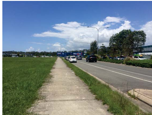
③ Approx. 2.5m wide concrete path and 900mm wide grass area between the kerb and the path
