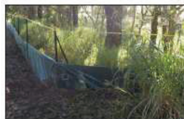
TREE PROTECTION & EROSION FENCE
