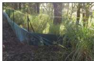
TREE PROTECTION & EROSION FENCE
