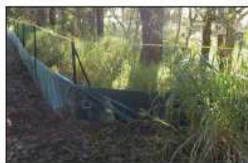
TREE PROTECTION & EROSION FENCE
