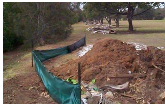
Plate 6-1 – Sediment Fences
