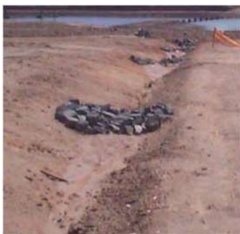
Plate 6-2 – Catch Drain
