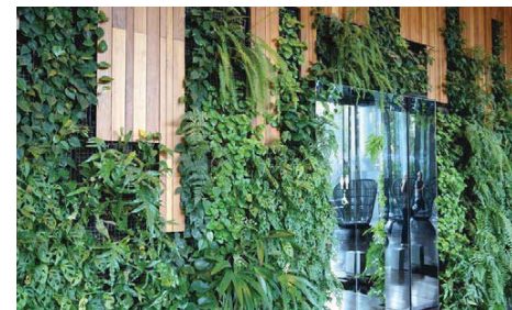
Green walls help soften architectural forms
