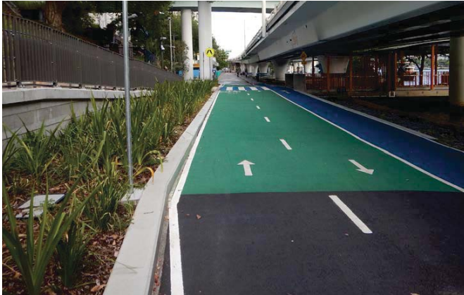
Figure 5.37: North Quay Existing Bikeway Conditions
