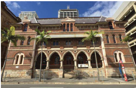
The Public Service Club and existing streetscape
