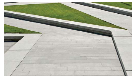
Use the level difference between the street level ground plane and the lower ground retail area to create new seating terraces
