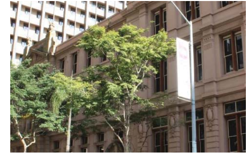
The Printery Building and existing streetscape
