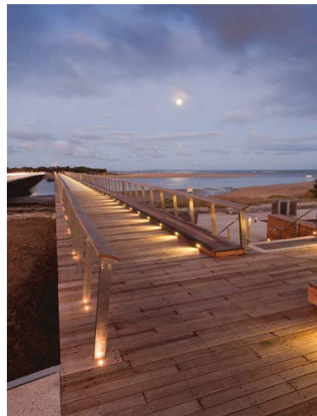
Lighting is an important element to maximise pedestrian safety
