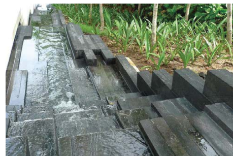
Utilise cascading water features at the Brisbane Steps to cool, and mask noise.
