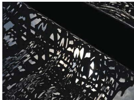
A vertical screen can conceal vehicle entry points
