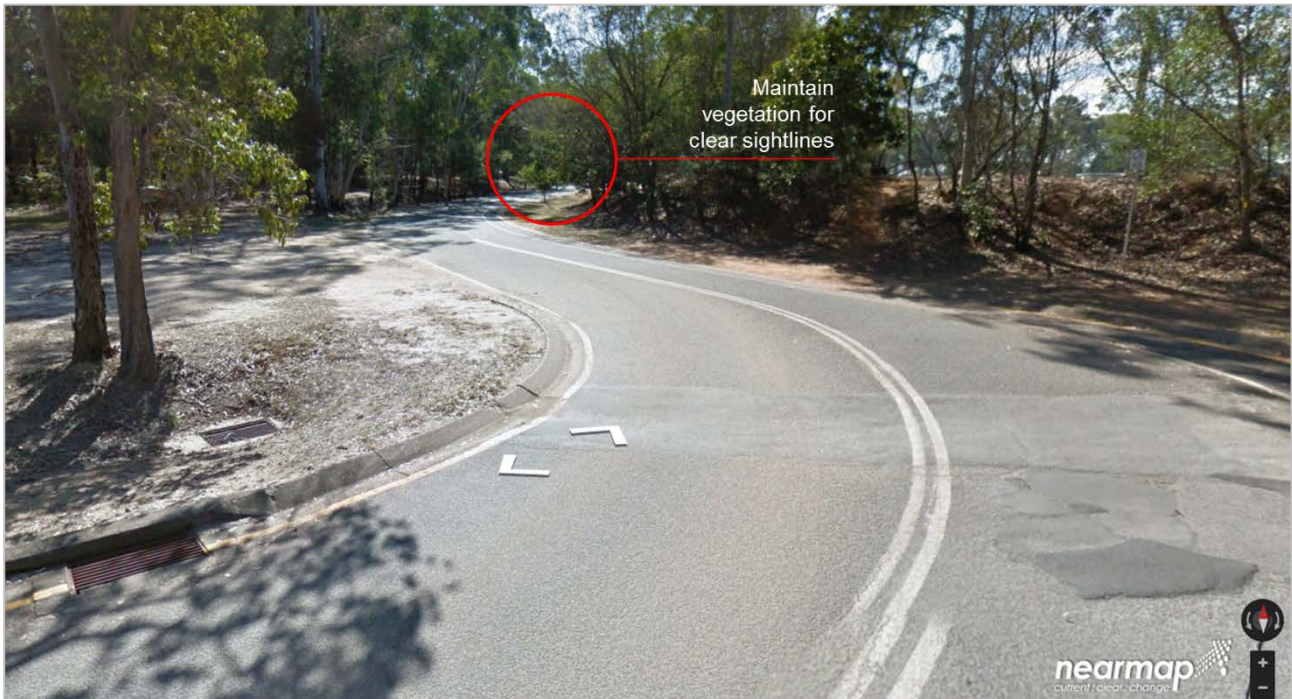
Figure 1-2 Existing Internal Road (view from right turning vehicle into temporary road looking north)
