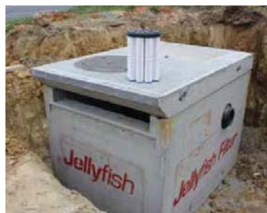
Kerb Inlet Jellyfish Filter is installed in a commercial development
