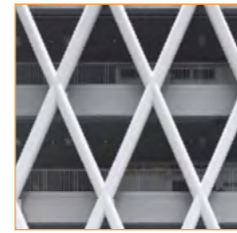
EXPRESSED STRUCTURAL STEEL
