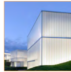
PUB ROOF STRUCTURE BEACON
