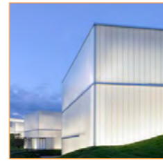
PUB ROOF STRUCTURE BEACON
