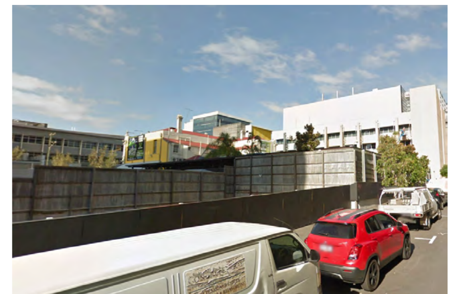
EXISTING BOUNDARY WALL ON BREWERS ST
