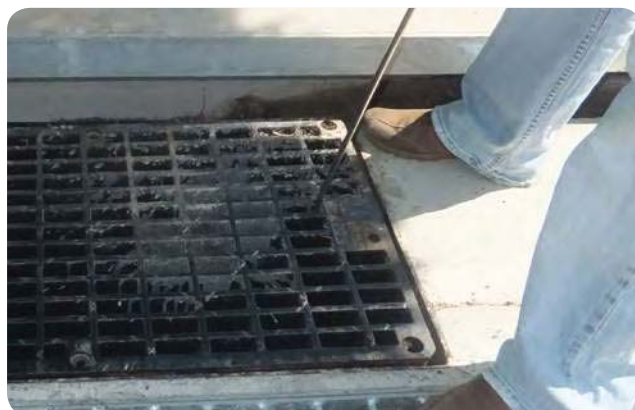
Photo 6 Insert hook near edge of grate
