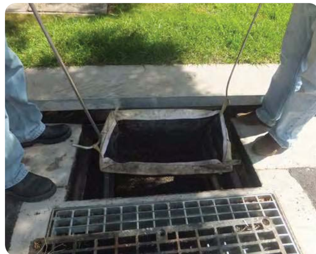
Photo 13 Lift the bag from the cage and support frame
