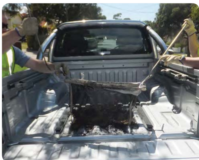
Photo 16 Grab the bottom lifting loops
