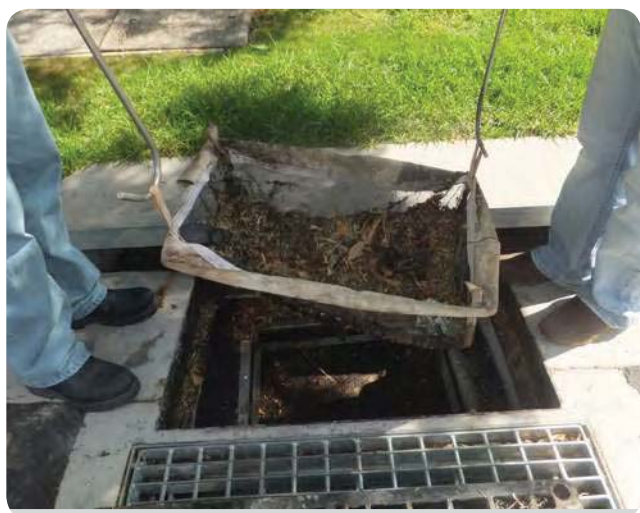
Photo 14 Lift the bag from the stormwater pit
