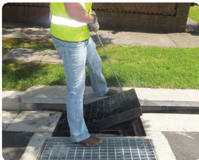
Photo 3 Lifting the grate
