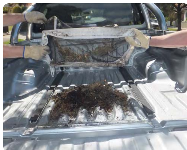
Photo 17 Lifting the bottom bag loops empty the filter bag
