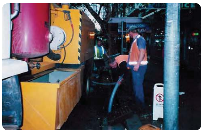
Photo 11 Cleaning an EnviroPod using the inductor method
