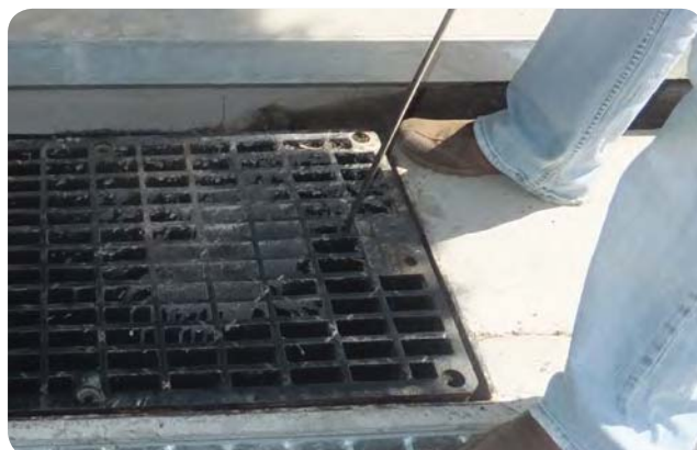
Photo 6 Insert hook near edge of grate
