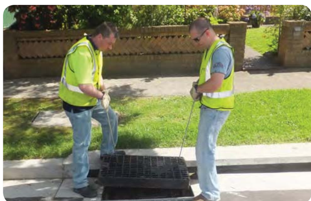
Photo 9 Lift grate above the support frame
