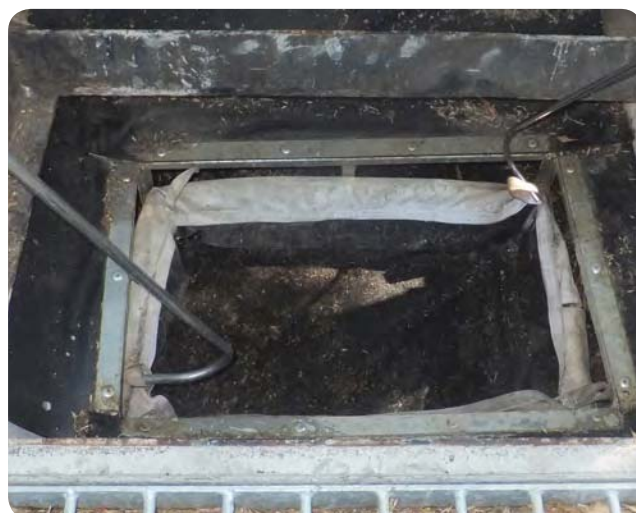
Photo 21 Correctly installed filter bag
