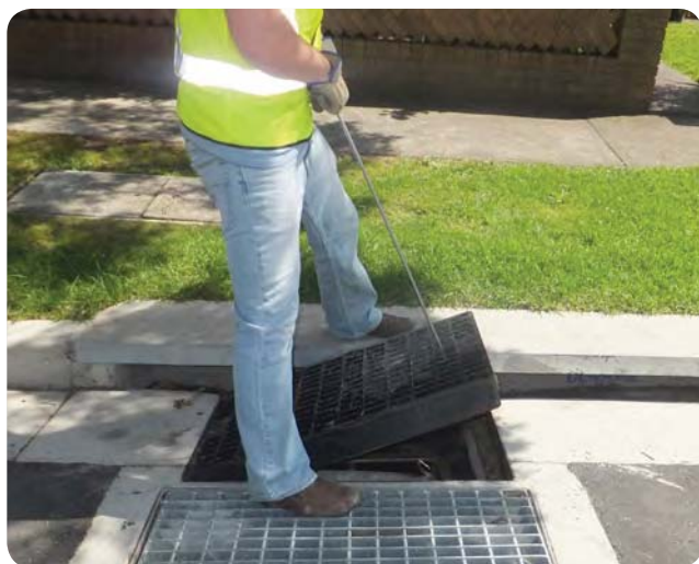
Photo 3 Lifting the grate
