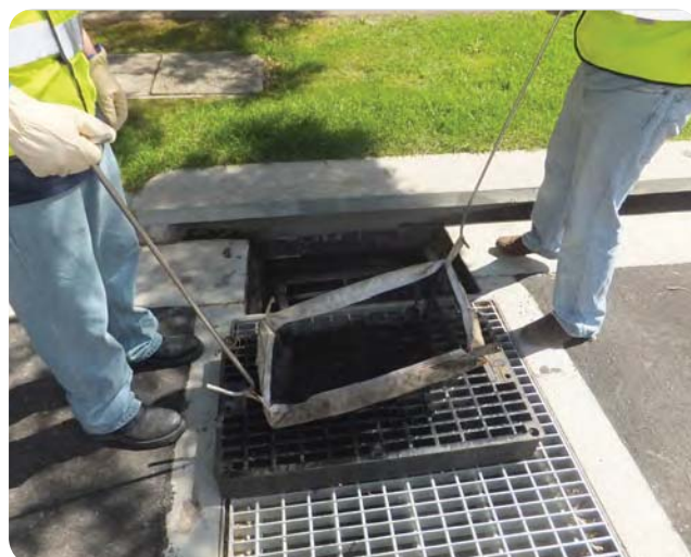
Photo 19 Reinstall filter bag
