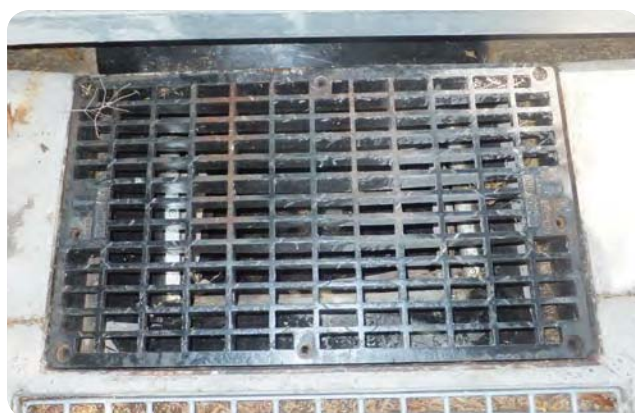
Photo 10 Reinstated non hinged grate
