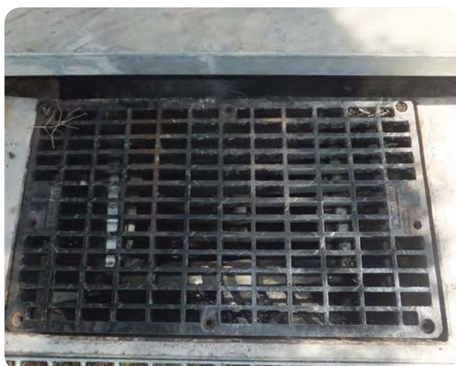
Photo 22 Installed filter bag and sealed pit
