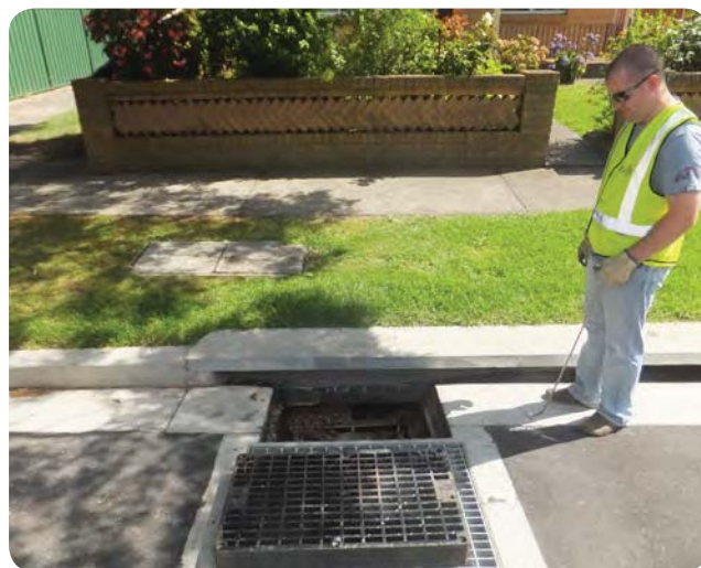
Photo 4 Fully open grate
