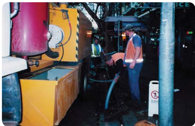
Photo 11 Cleaning an EnviroPod using the inductor method
