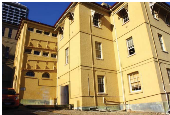
Figure 16 – Northern elevations of Building viewed from Queens Wharf Road
