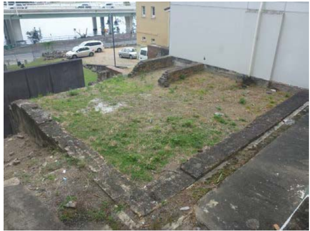
Figure 12 – Remains of 1916 addition to Building viewed from William Street Level
