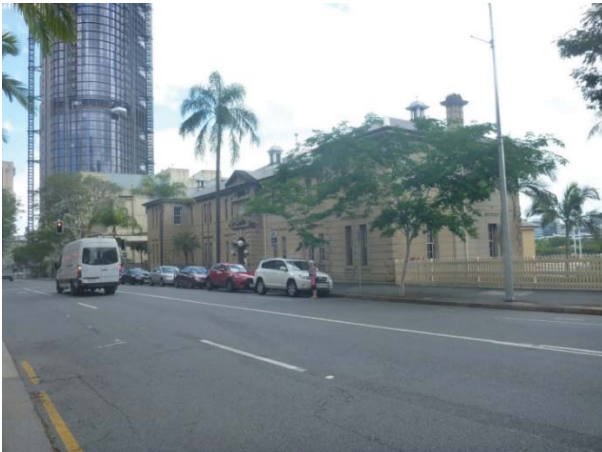
Figure 13 – View of Building along William Street from the North
