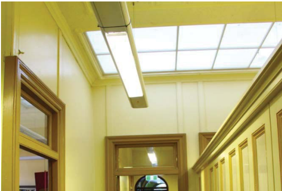
Figure 23 – Skylight Above Central Corridor
