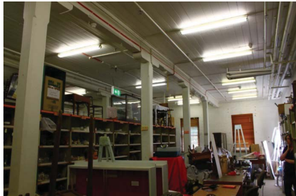
Figure 24 – Basement in Queens Wharf Road Wing
