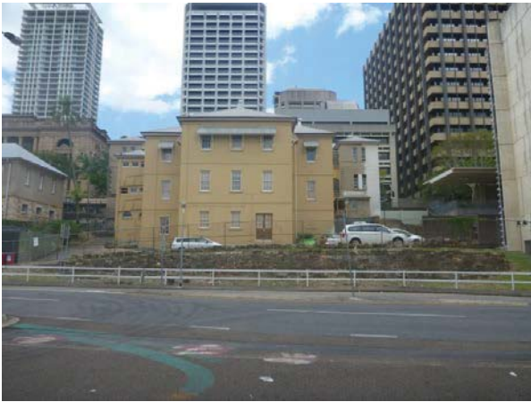
Figure 11 – View from Queens Wharf Road of Rear Wing
