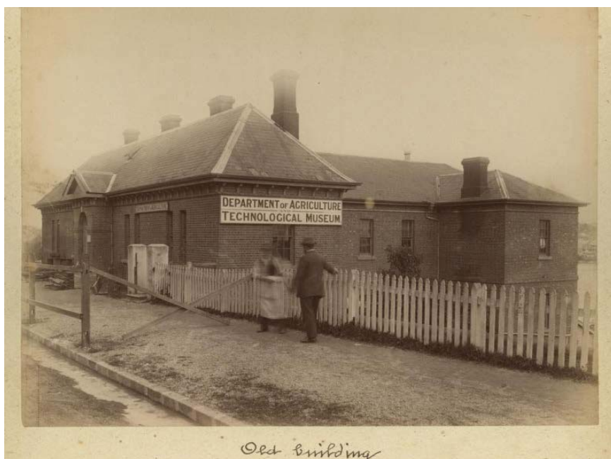
Figure 4 – Former DPI Building c1890
