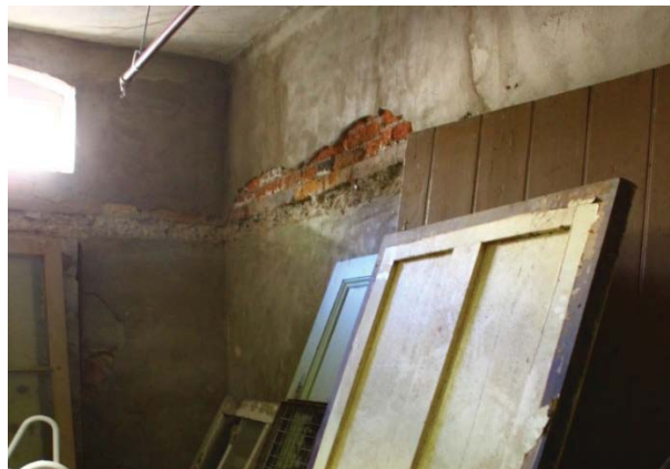
Figure 26 – Storage Room on Southern side of Sub-Basement
