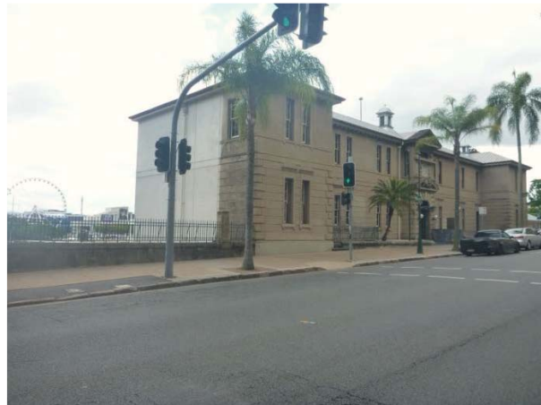
Figure 14 – View of Building along William Street from the South
