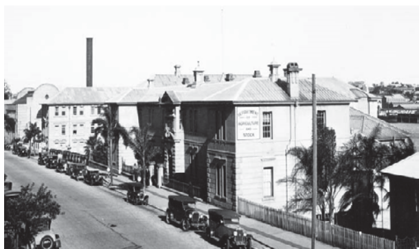
Figure 7 – William Street Elevation of Former DPI Building, 1936
