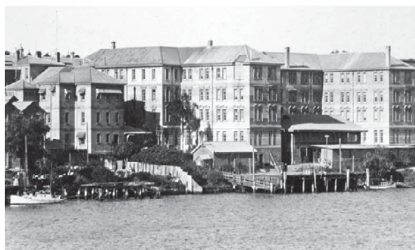
Figure 8 – Queen's Wharf Elevation of Former DPI Building Showing Southern Extensions to the Building, 1938
