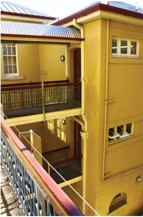
Figure 17 – 1924 Toilet Block to the Rear of the 1860s Building
