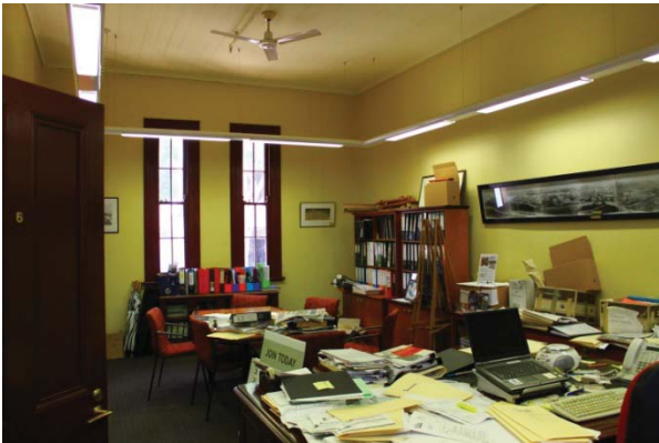
Figure 18 – Typical Ground Floor Office Fitout with Timber Ceiling, Carpeted Floors and New Services
