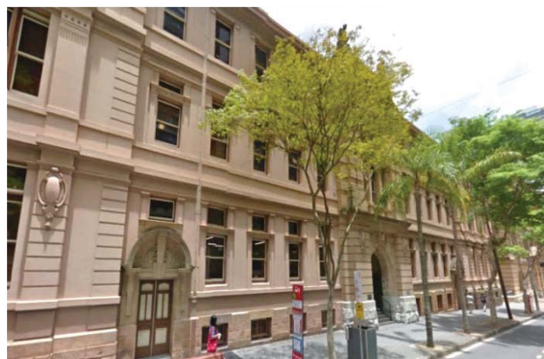
Figure 24 - George Street Elevation, looking towards the Central Entrance
