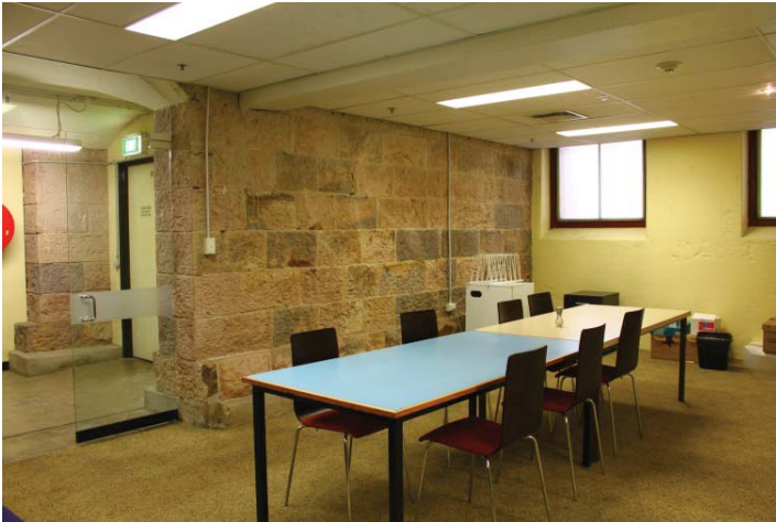
Figure 29 - Basement Showing Stone Wall
