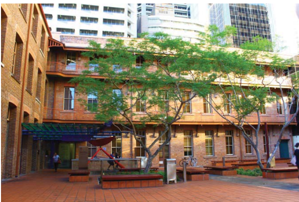
Figure 23 - George Street Building Viewed from Courtyard
