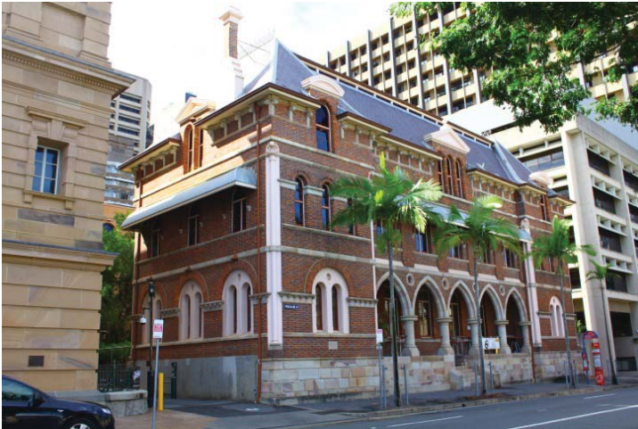
Figure 16 – William Street Façade
