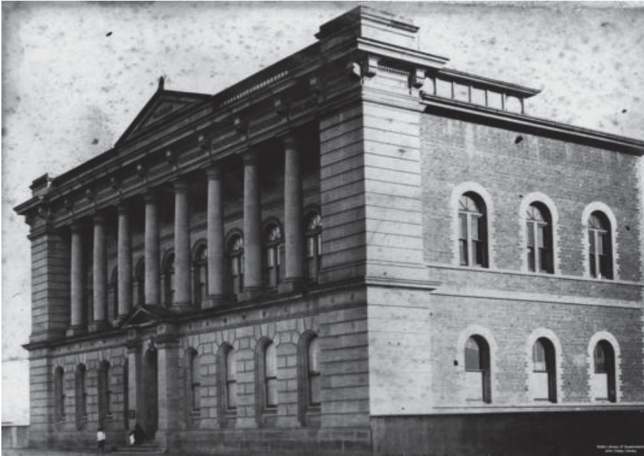
Figure 3 – The original Museum building constructed in 1876-79. Note the face brick side elevation and original clerestory to the roof top
