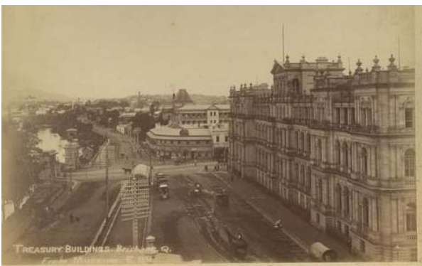
Figure 11 – William Street and Treasury Building, 1906
