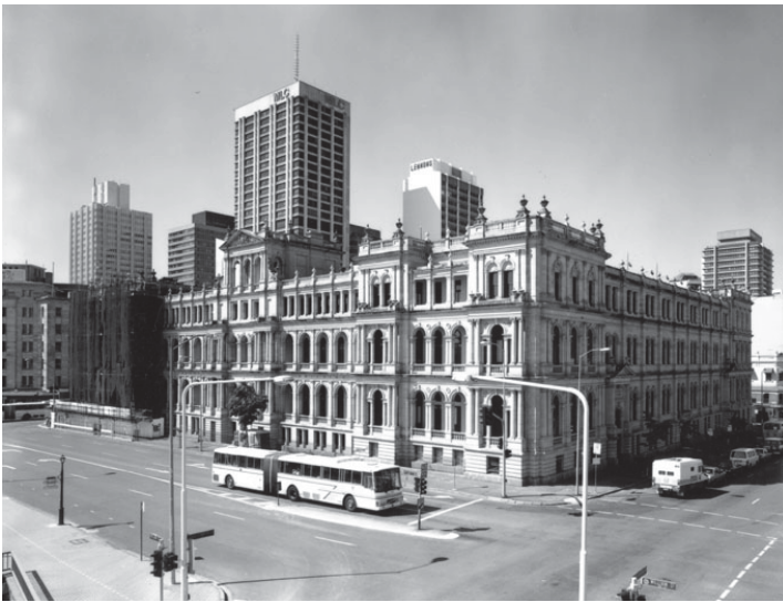
Figure 15 – Treasury Building, Queen/William Street Corner, 1991
