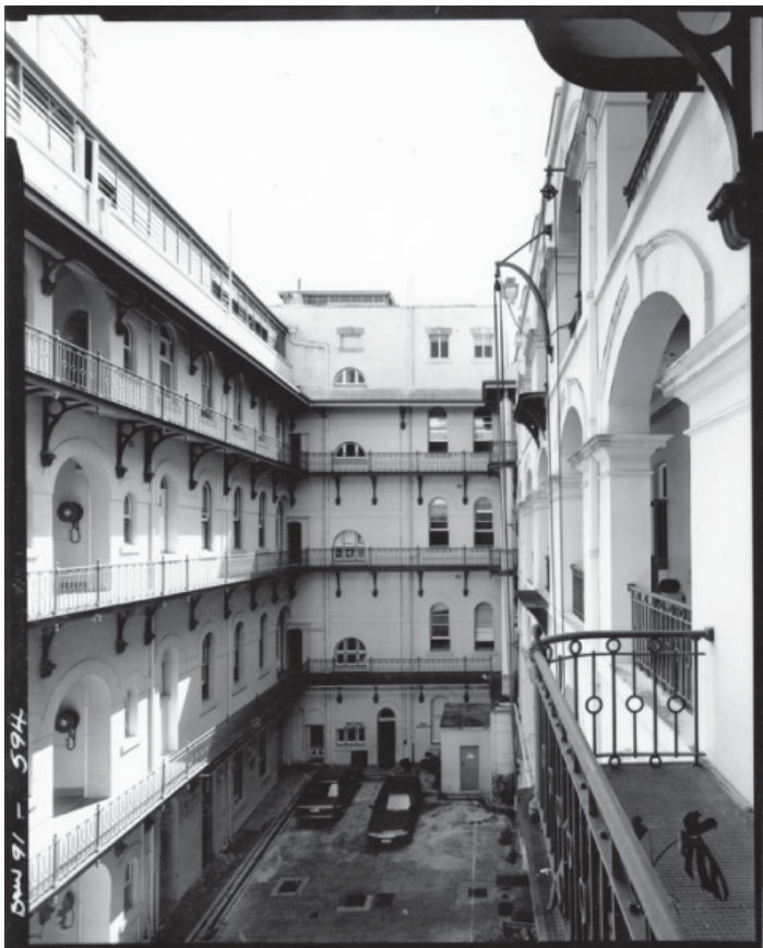
Figure 27 – Courtyard in 1991, prior to Casino adaptive reuse works
