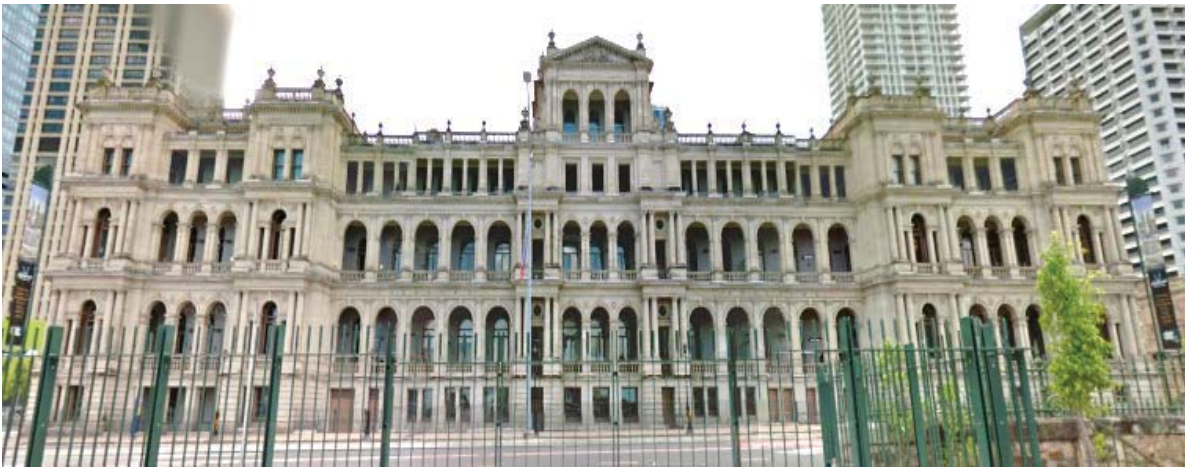
Figure 24 – Arcaded South-Western Façade, with central pediment and pavilions
