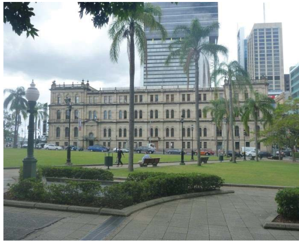
Figure 28 – View across the gardens to the former Treasury Building
