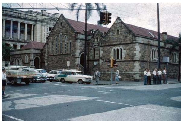
Figure 6 – Former Diocesan buildings at the site in the early 1960s
