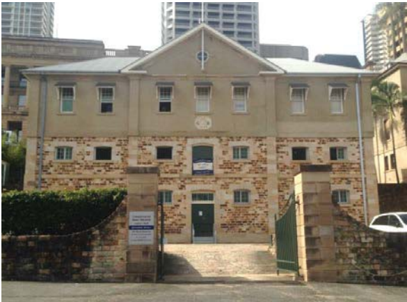
Figure 26 – Queens Wharf Road elevation Source: Urbis 2016
