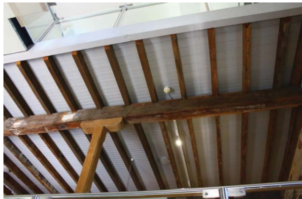
Figure 31 – Underside of Timber Floor
