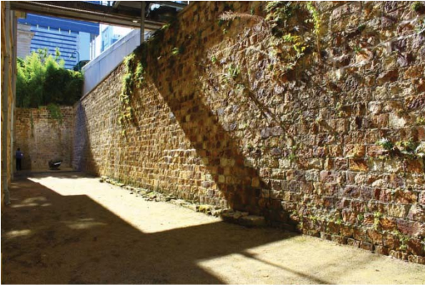
Figure 23 – William Street retaining wall
