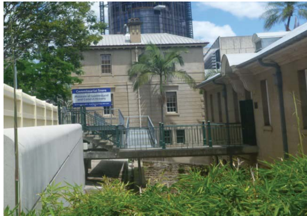
Figure 27 – Gangway and steel ramp Source: Google Earth
