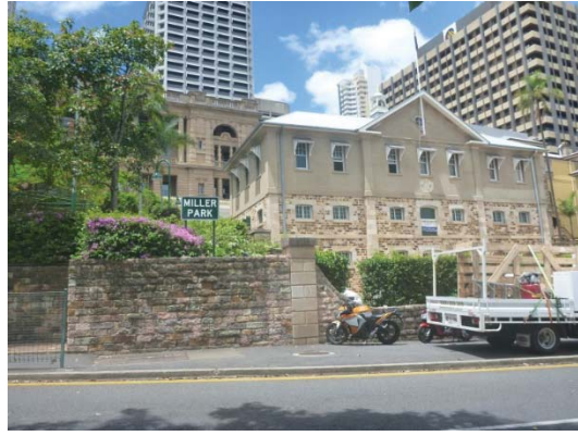
Figure 24 - Queens Wharf Road retaining wall, extending to Miller Park
