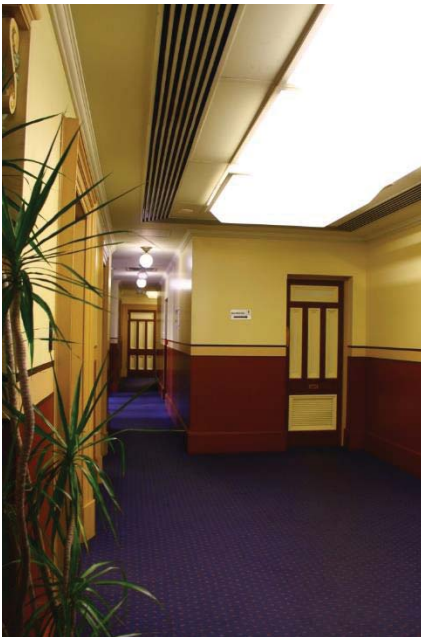
Figure 26 – Hallway with suspended ceiling and lift lobby
