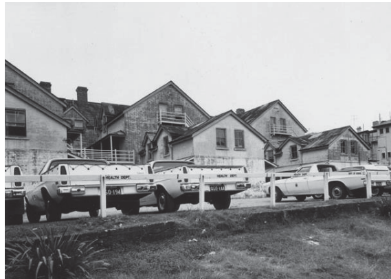
Figure 13 – Rear of The Mansions, 1973
