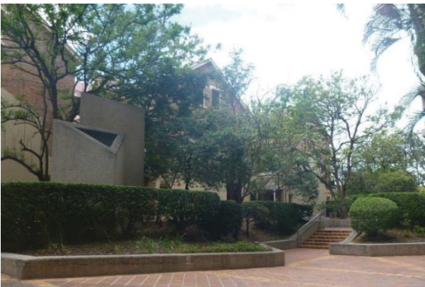
Figure 16 – Rear of The Mansions
