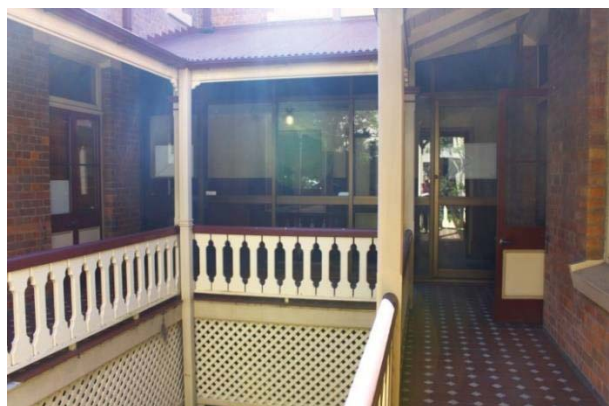
Figure 20 – Reconstructed verandah, First Floor
