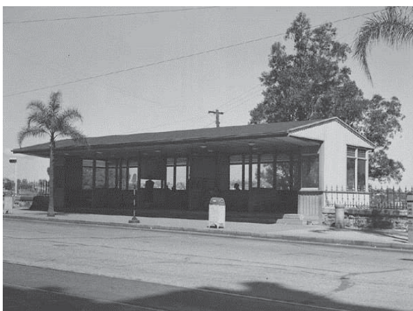
Figure 6 – Bus Shelter in 1950
