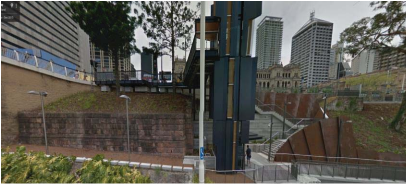
Figure 10 – Lift adjacent to Bridge Abutment, December 2015
