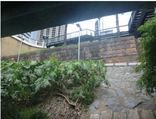
Figure 16 – Victoria Bridge abutment from Bicentennial Bikeway
