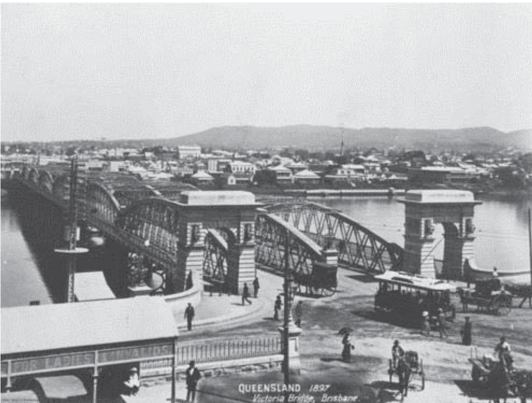
Figure 9 – Victoria Bridge, 1897. Abutment remnants of that at left of bridge.
