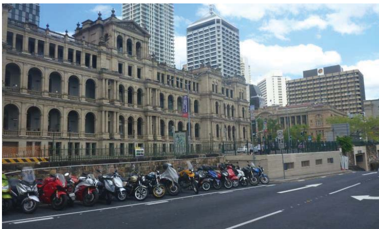
Figure 12 – William Street retaining wall
