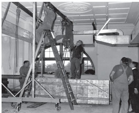
Figure 10 – Works Inside the Camera Room, 1970
