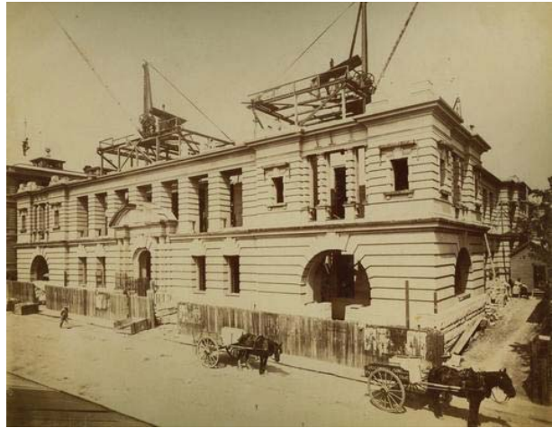
Figure 4 – Construction of the Building, 'Land and Survey Office', 1902
