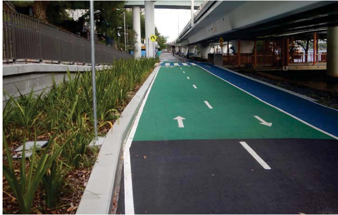
Figure 5.37: North Quay Existing Bikeway Conditions
