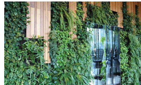
Green walls help soften architectural forms
