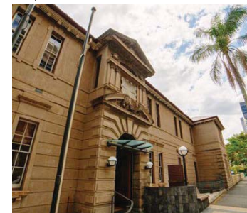
Former DPI Building entrance
