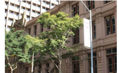
The Printery Building and existing streetscape
