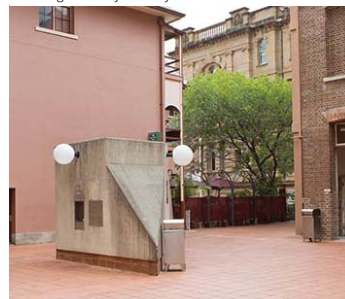
Existing Public Service Club courtyard
