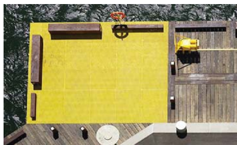
New constructed edge structures are intended to evoke the history of the working operation of wharves in this area
