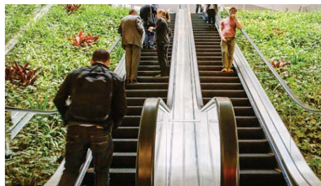
Install tree and planting in the lower ground retail area
