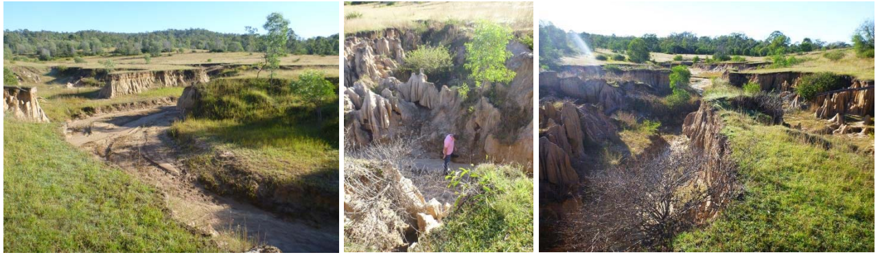
Examples of eroded drainage paths in the upper to mid catchments
