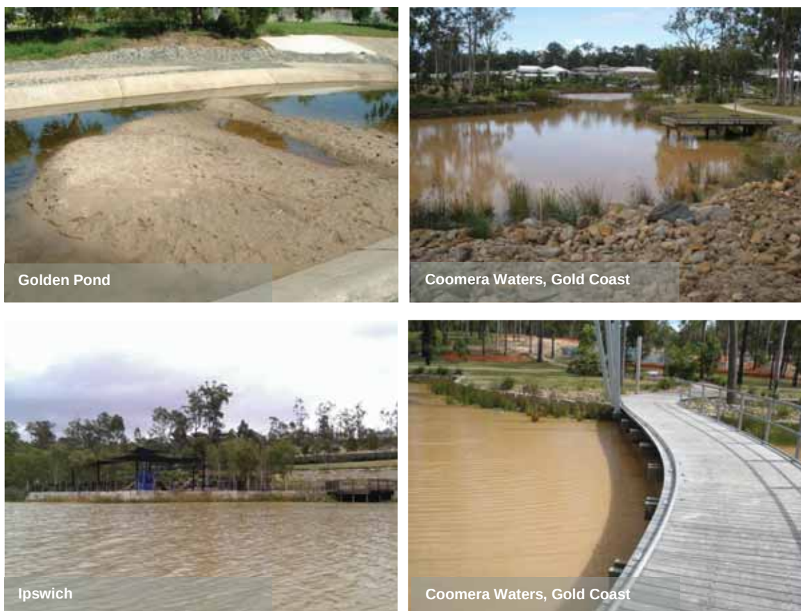
Figure 4-8 Examples of Excessive Sediment Accumulation and High Turbidity in Waterbodies
