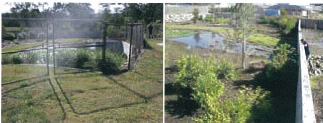
Figure 4-2 Example of a Poorly Integrated 'End-of-Pipe' Bioretention Basin
