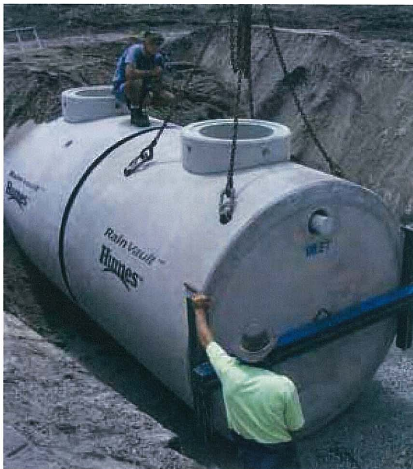
Figure 3-10 Installation of an Underground Stormwater Harvesting Tank
