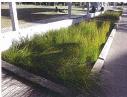
Example of Rain Gardens
