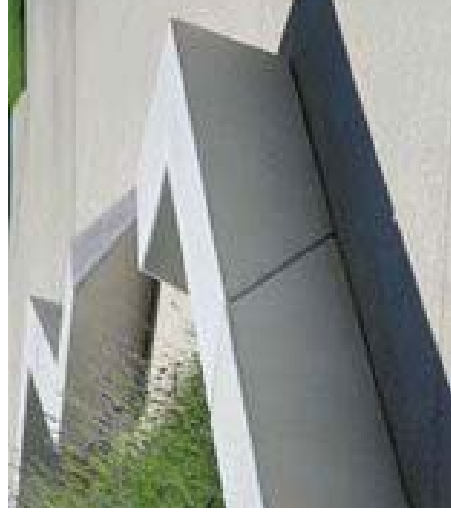
Cast insitu concrete seats
