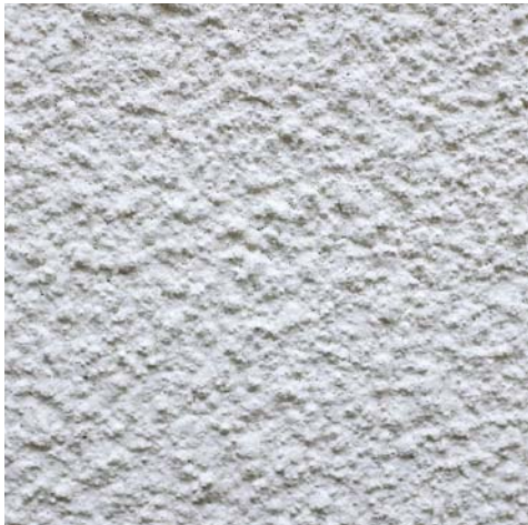
TEXTURED CONCRETE RENDER
