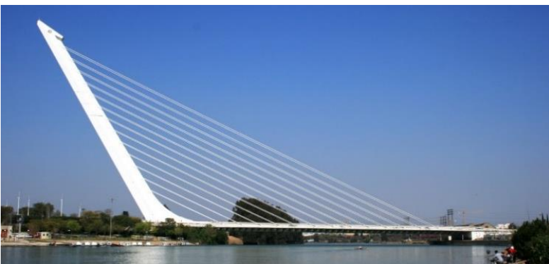
FIGURE 12 - PRECEDENT IMAGE: ALAMILLO BRIDGE – SEVILLE, SPAIN SINGLE MAST. MAIN SPAN = 200M. HEIGHT OF MAST = 140M (DATUM UNKNOWN)
