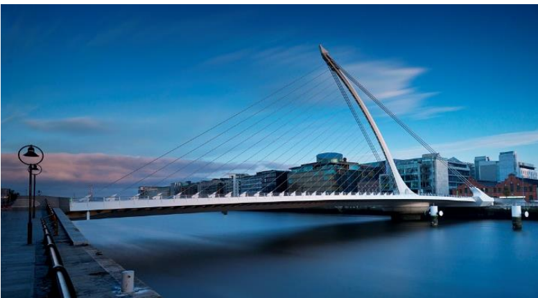
FIGURE 11 - PRECEDENT IMAGE: SAMUEL BECKETT BRIDGE – DUBLIN, IRELAND SINGLE MAST. MAIN SPAN = 95M. HEIGHT OF MAST = 46M (ABOVE MWL)
