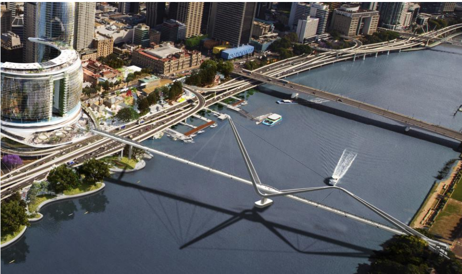
FIGURE 10 - CURRENT PROPOSAL NEVILLE BONNER BRIDGE ARCH + MAST HYBRID. MAIN SPAN = 145M. HEIGHT OF MAST = 77M (ABOVE HAT)
