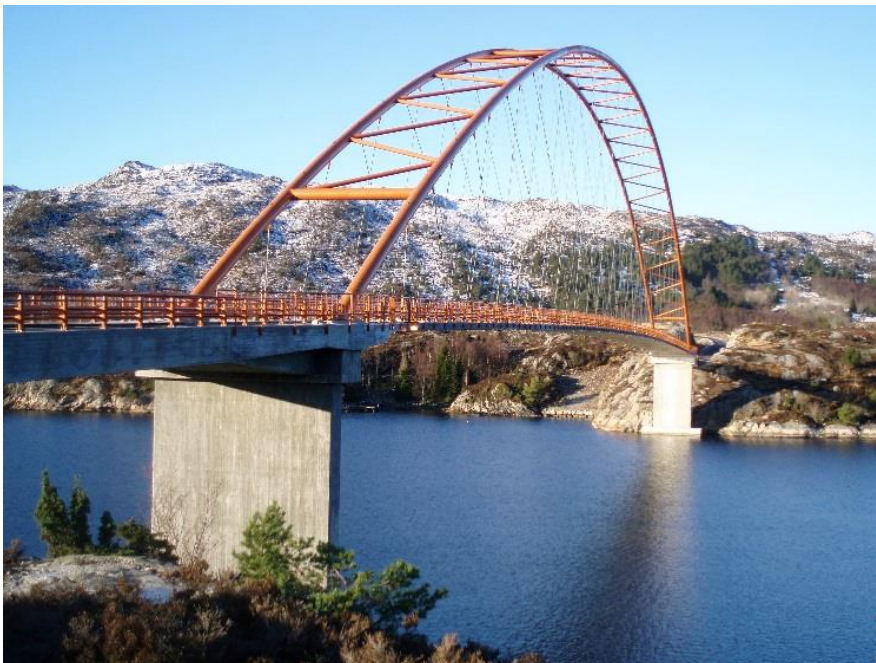
FIGURE 13 - PRECEDENT STUDY: BRANDANGER BRIDGE - BRANDANGER, NORWAY NETWORK ARCH BRIDGE. MAIN SPAN = 220M. HEIGHT = 37.4M (ABOVE DECK)
